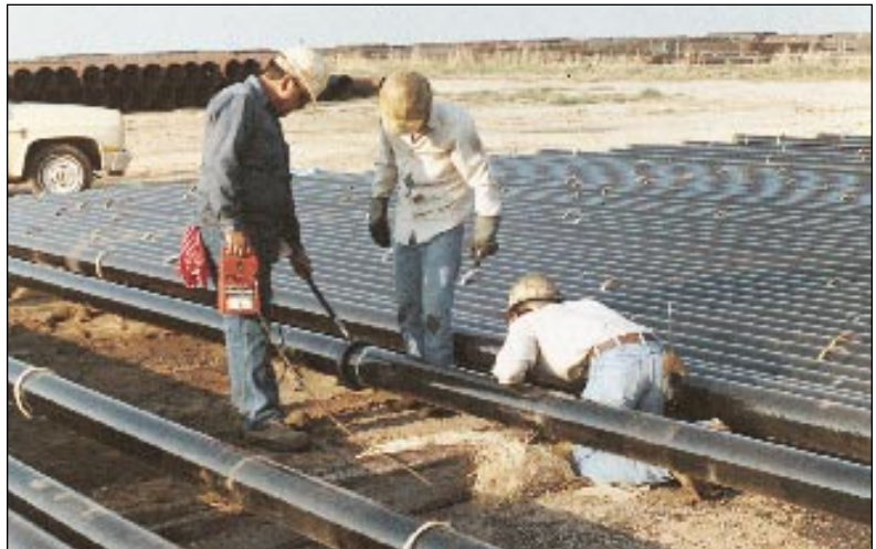
Fig. 4 - Holiday testing can be performed as soon as one hour after application of a 100% solids plural component polyurethane coating.
