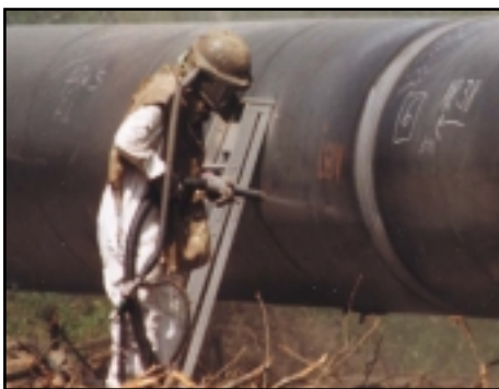
On site surface preparation of the welded steel pipe joints
