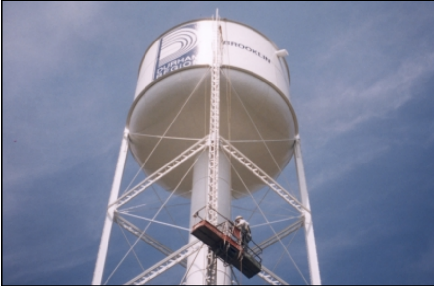
The Brooklin water tower was repaired using Madison's Corroccote II PW.
