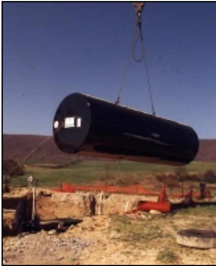
Installing FibreThane ACT-100-U® underground tanks.
