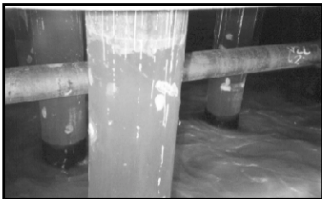
Steel pipe pilings coated with Madison's Corropipe II TX-15: very little damage after 5 years of service.
