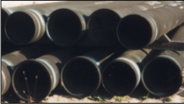
Installation of lined and coated Ductile Iron Pipe in San Diego.
