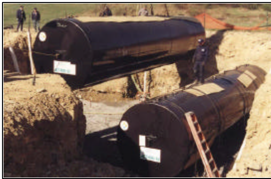
Figure 2 Installation of the STI ACT-100-U ® Tanks
