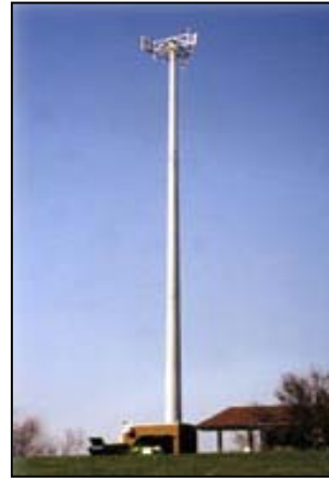
Figure 10. A 100% solids, rigid, aliphatic polyurethane coating used for protection of a communication tower
