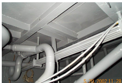
Figure 13. The ballast tank was coated with a 100% solids rigid polyurethane coating
