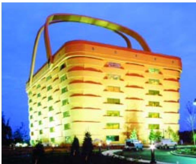
Architects built this suburban Ohio office building to resemble the baskets manufactured by its owner. Painting the galvanized structural steel completes the realistic effect and provides superior corrosion resistance.
