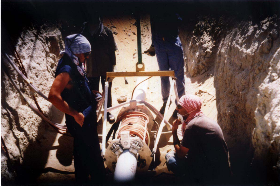
FIGURE 7. Application of magnetic induction heat to a pipeline joint in the desert.
