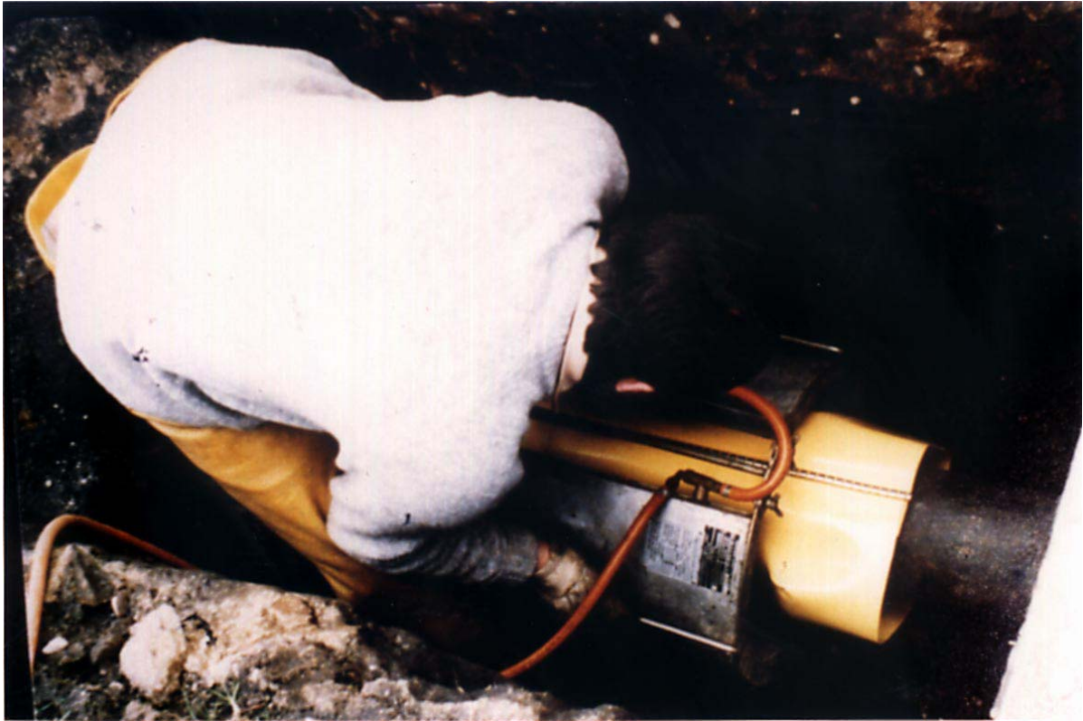
FIGURE 3. A polyethylene heat shrink sleeve being heated into shape by magnetic induction heating (photo courtesy of Shaw Industries).
