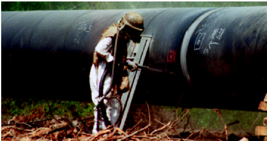
Figure 5. Field joint coating with polyurethane
